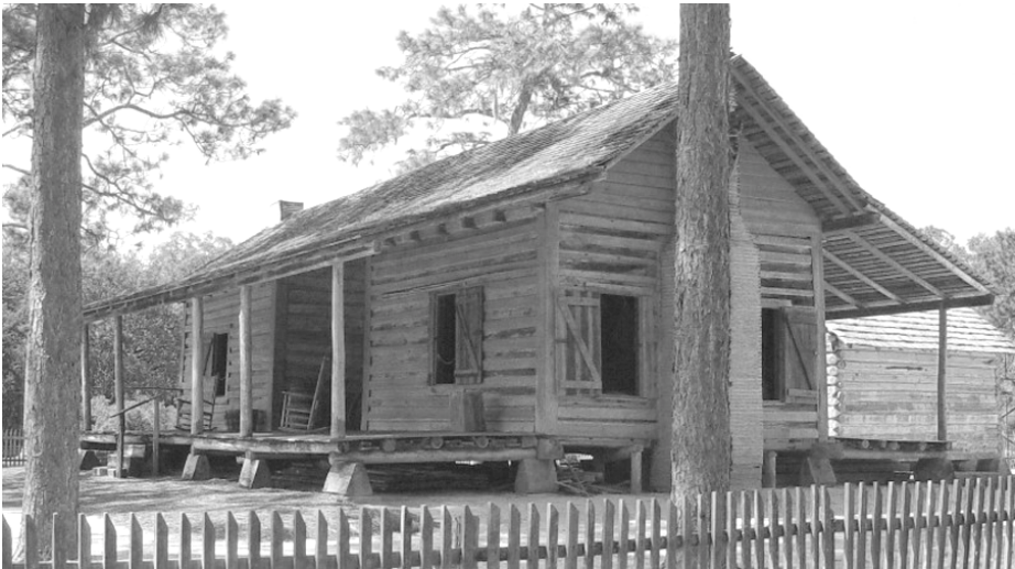
Figure 1: Typical Florida Cracker House Source: (Forest Capital State Museum 2010)
