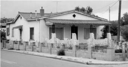
Figure 12 Residence at 707 Agua Fria Street
