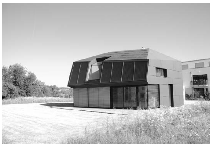
Haus der Zukunft, 2009 Regensburg, Germany New single-family house 175 m 2 Picture: Gitte Gylling
