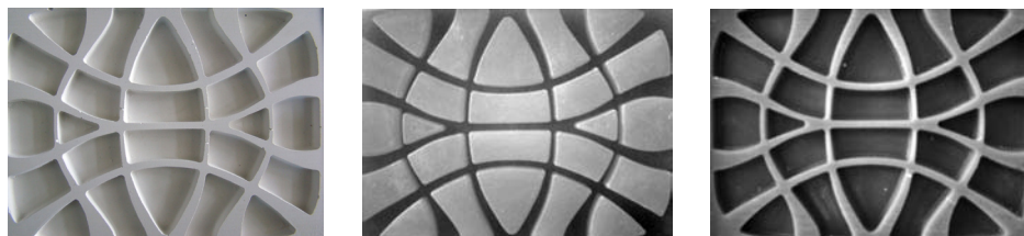
Figure 3 a,b,c: Nervi's work demonstrates a strong correlation between aesthetics, statics, materials and construction technology. This is evidenced in the mezzanine slab in the Palazzo dello Sport and the Gatti Wool factory. These have been studied to gain tangible insight into Nervi's intuition and working method.
