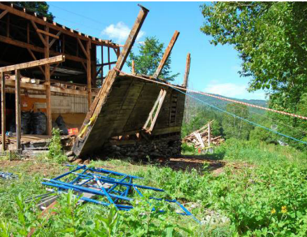
Photo 4: Back wall being removed by group effort
