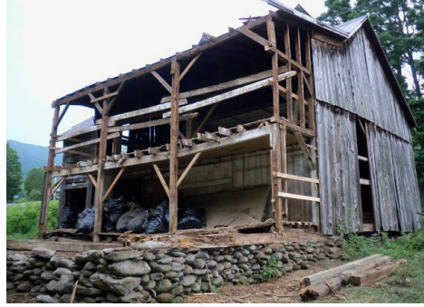
Photo 5: Main element after removal of secondary element
